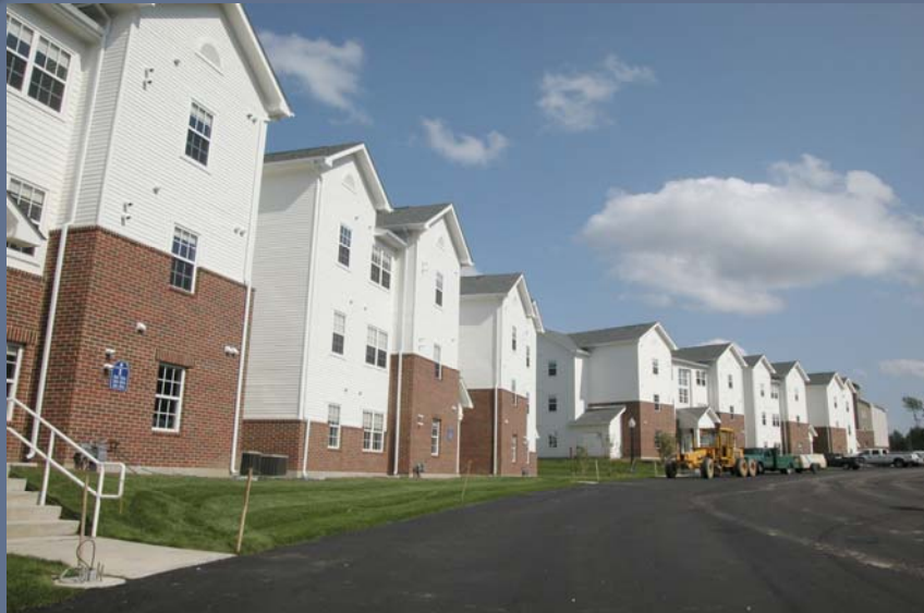
North Campus Renovation (Charter Oak Apartments)
