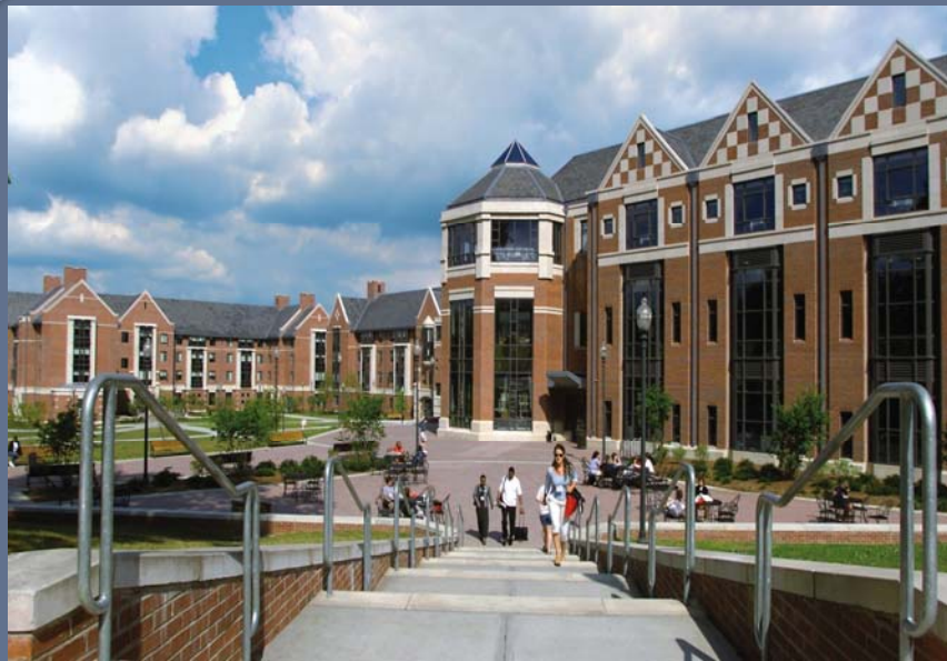
South Campus Complex
