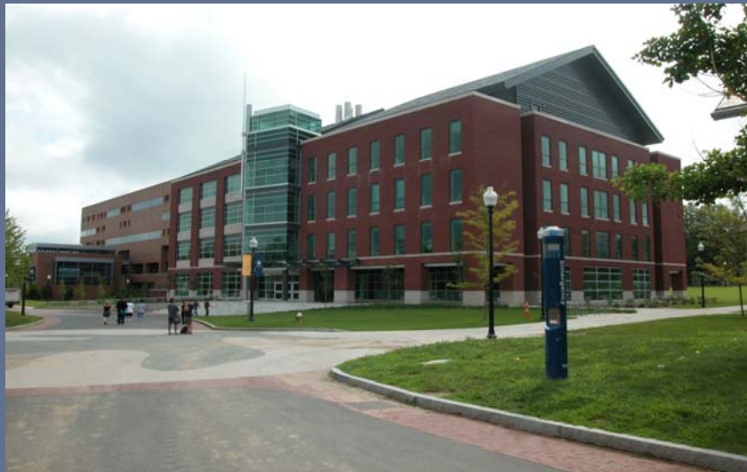
Technology Quadrant Phase II (Information Technology Engineering Building)
