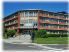
Monteith Building Renovation
