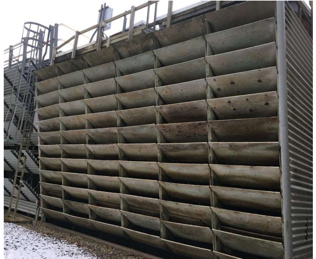
Plywood Cooling Tower Cell
