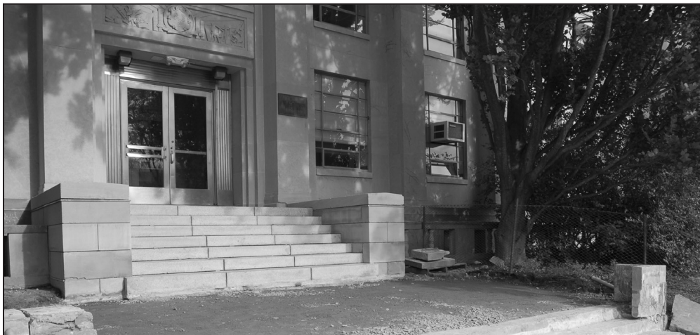
THE W. B. YOUNG BUILDING, HOME OF THE COLLEGE OF AGRICULTURE AND NATURAL RESOURCES, WAS BUILT IN 1953 AND IS SCHEDULED FOR A FULL RENOVATION AND, POSSIBLY, AN ADDITION. THE RENOVATION WORK HAS BEGUN, AND WILL INCLUDE WINDOW REPLACEMENT, REPOINTING MASONRY, RESTROOM RENOVATIONS, AND UPGRADING THE MECHANICAL SYSTEMS. REPLACING THE MAIN STAIRWAY WAS ONE OF THE FIRST JOBS.
