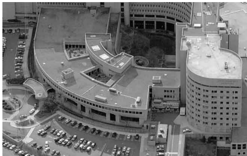
UHC Clinic Building
