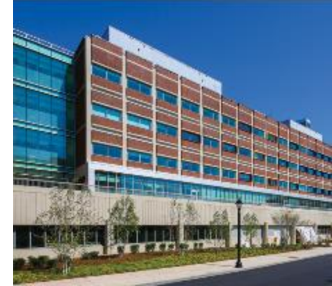
Gant Building Renovation Phase I-II
