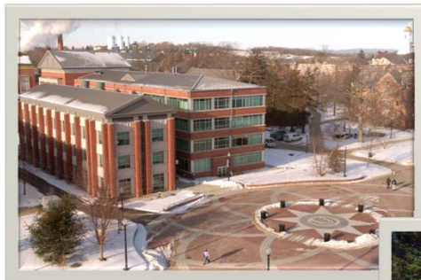
Business School Renovation (Rowe Center for Undergraduate Education): Completed in 2004
