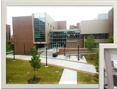
Psychology Building Renovation & Addition: Completed in 2013
