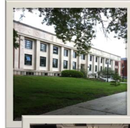
Young Building Renovation: Completed in 2015
