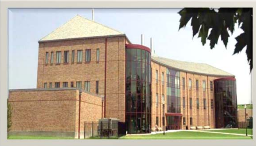
Agriculture Biotechnology Facility: Completed in 1999 & 2002
