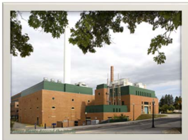
Heating Plant Upgrade (Cogeneration Facility): Completed in 2006
