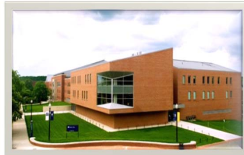
Student Union Addition: Completed in 2006
