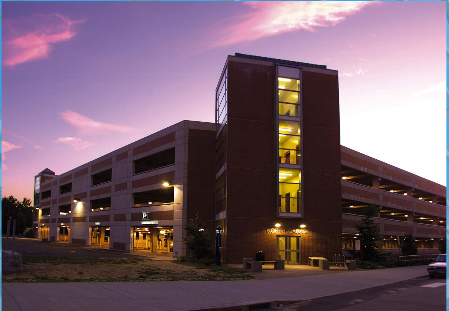
North Parking Garage
