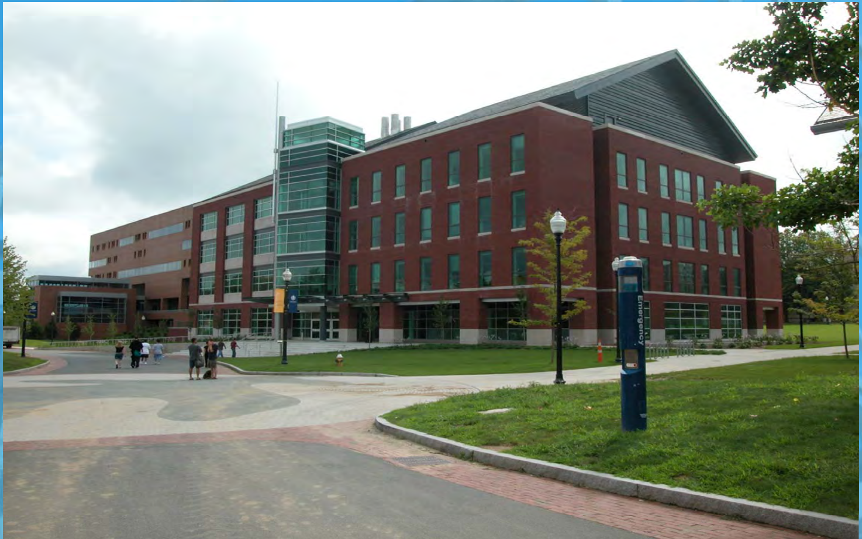
IT Engineering Building
