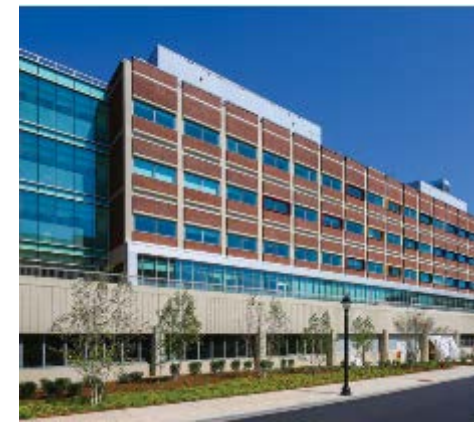
Gant Building Renovation Phase I-II
