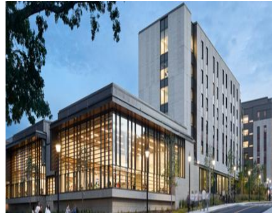
Connecticut Residence Hall
