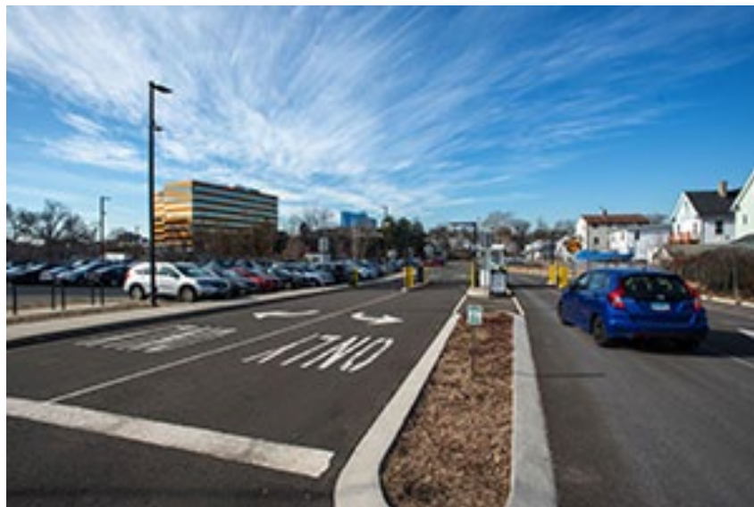
New Stamford Parking Lot- Abutting Properties to the right side
