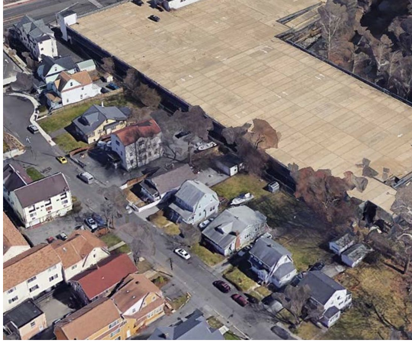
Vernon Place prior to Garage Demolition and Remediation Projects
