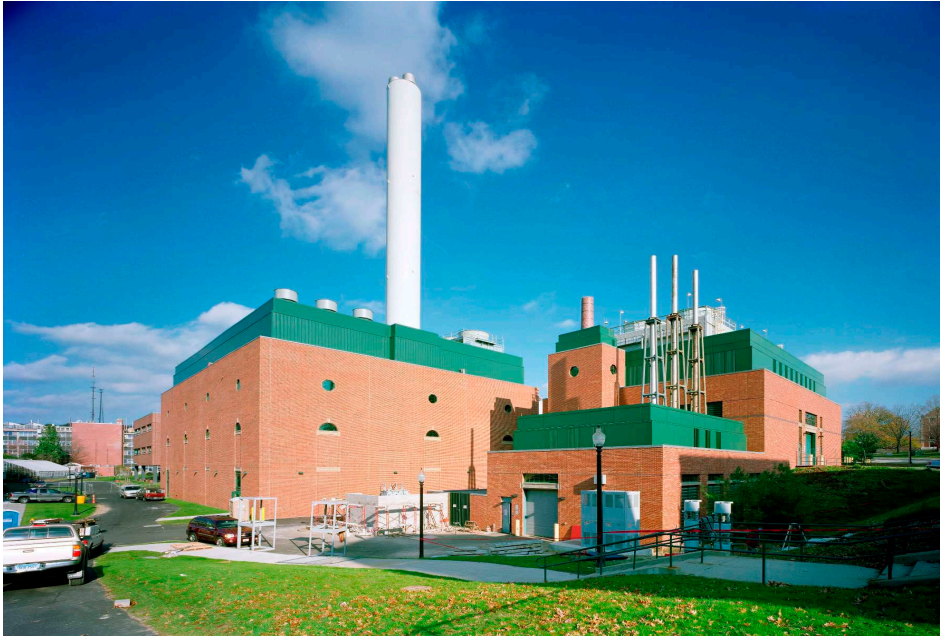
Existing Central Utility Plant
